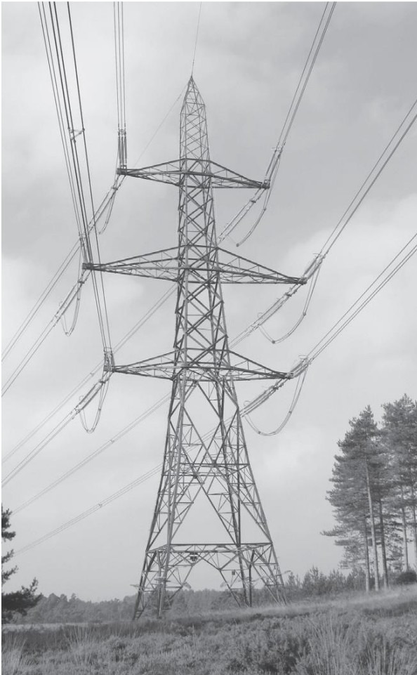
Photo 2: Deviation nest pylon with top entry boxes
